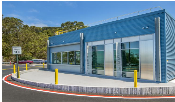
FLEXLAB is capable of rotating up to 270 degrees to simulate solar conditions.
